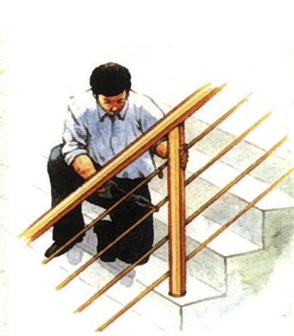
Twist in-fill (filler) to suit Stair angle
